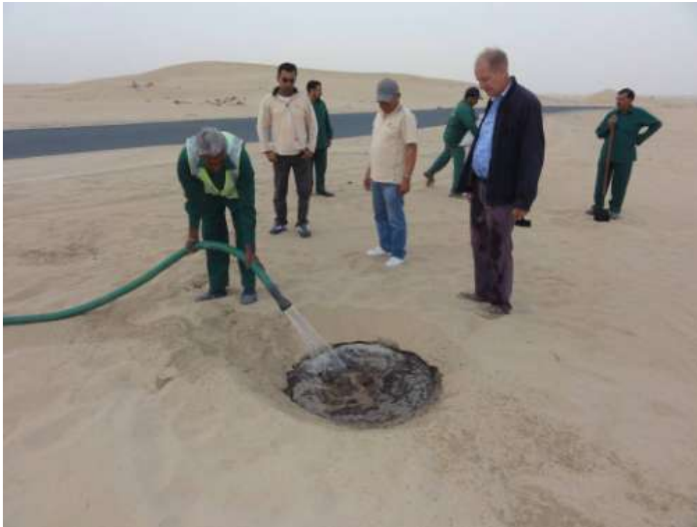
Creating the capillary column by adding 40 liters of water in the planting hole
